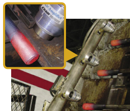
Model 6042 2" (51mm) Adjustable Air Amplifiers with swivel fittings cool inductively heated axles prior to installing the hubs.
